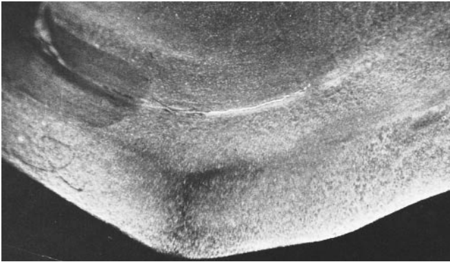
FIGURE 7. Fluorescent indication of crack in foot of toilet bowl.
