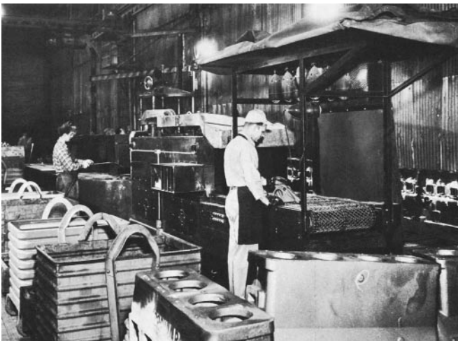
FIGURE 6. Mechanized liquid penetrant testing of castings in tractor factory.
